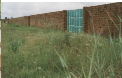
Completed wall and gate
